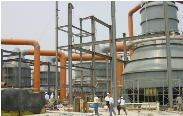
Installation of NaCl/Na 2 SO 4 combined plant
